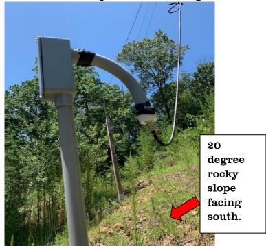
Modified drop using a 90 degree sweep to simplify construction and easier to pull the coax through.
